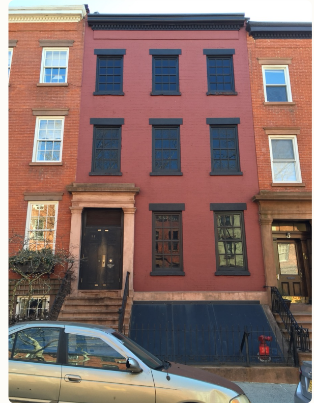
a subway vent behind a townhouse facade
